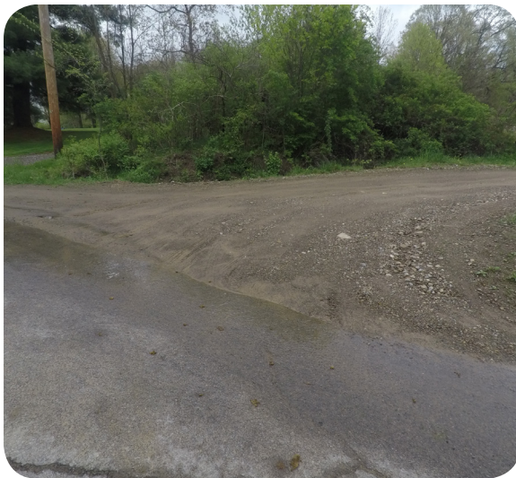
McCracken Road Washout Issues
