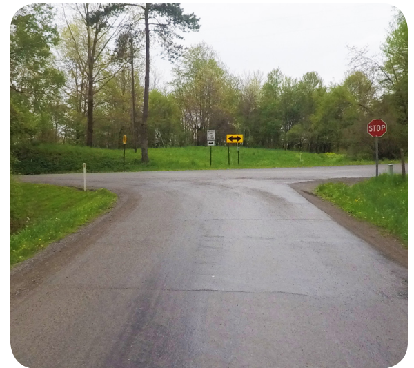
Intersection of Fryermuth & Tamarack Roads
