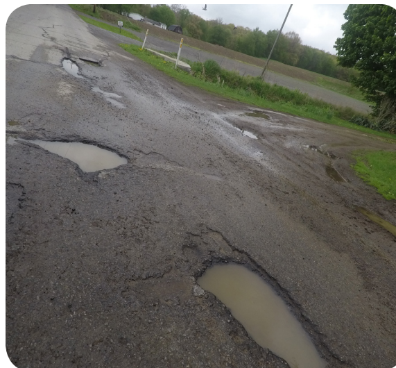
Schreck Road Surface/Drainage Issues
