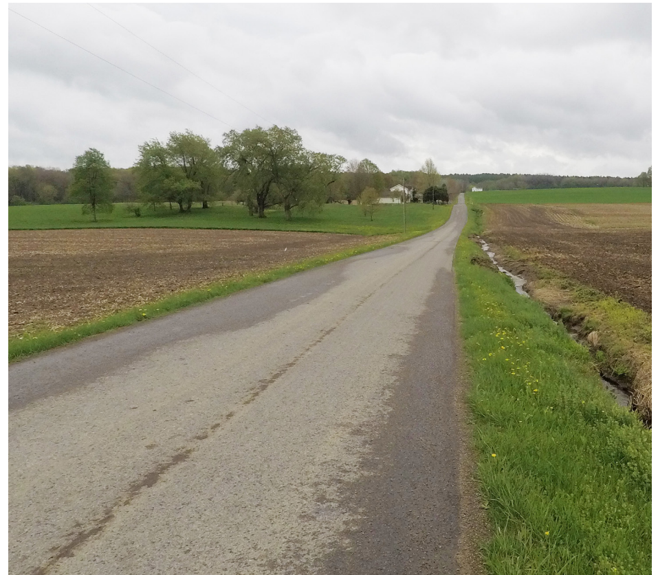
A Typical Township Roadway
