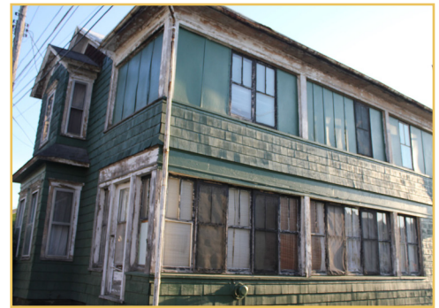
Peeling paint, rotting siding and broken windows at a house in Meadville.
