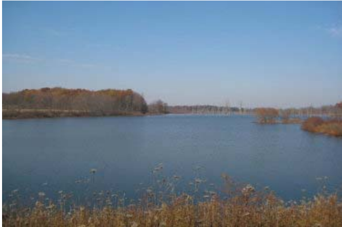
Photo taken from atop dam, facing north toward lower reservoir
